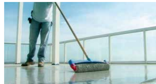
Deck Polyurea FFP Brush applied, hybrid polyurea membrane system
