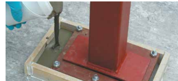
Deck Plug Fast setting cementitious plugging compound
