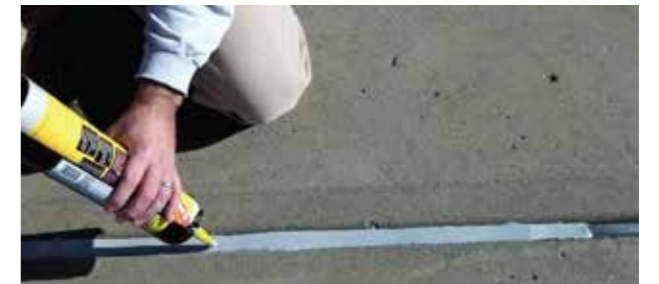
Seal Strong Semi rigid polyurea sealant
