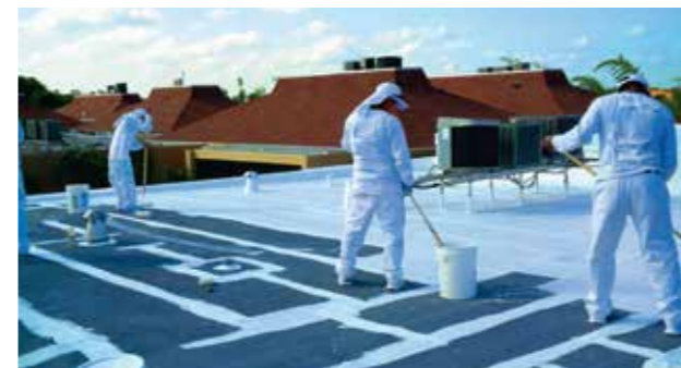
Deck Proof High build, flexible acrylic membrane system
