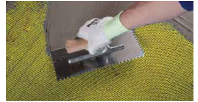
Deck Elastic M Cementitious elastomeric membrane system
