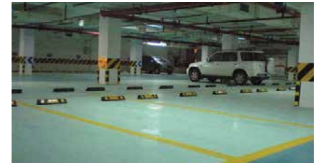
Deck Floor PU Solventless heavy duty polyurethane floor coating
