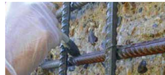
Deck RHAB Mineral corrosion protection coating
