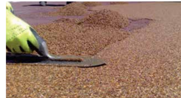
Pervipave RB Resin bound pervious paving
