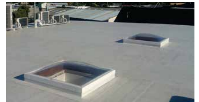
Deck PU-1K Single component, moisture cure polyurethane system
