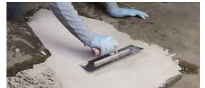
Deck Repair EP High strength epoxy repair
