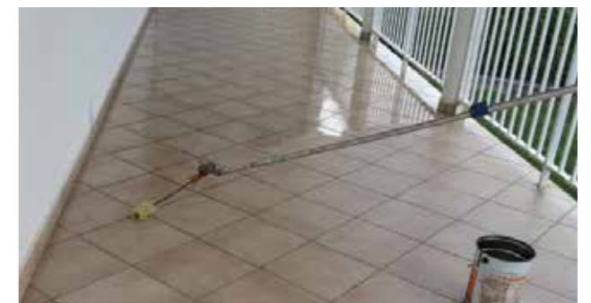
Deck PU Trans Aliphatic polyurethane concrete sealer
